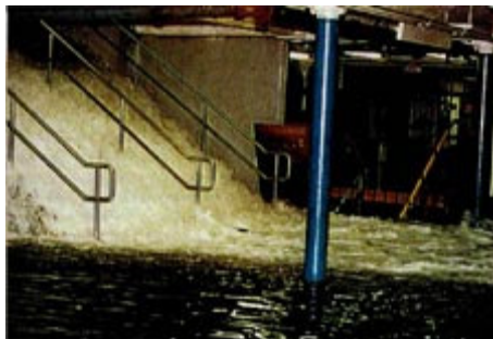
PATH station in Hoboken during a 1992 nor'easter. (Source: Metro New York Hurricane Transportation Study, 1995).
